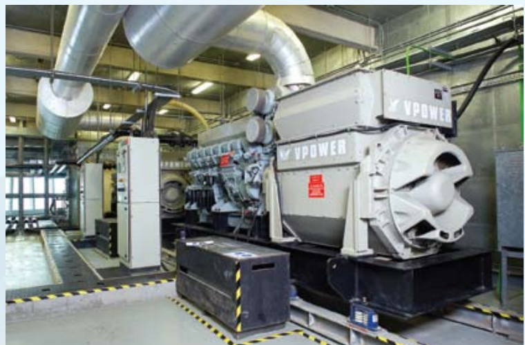
One of the High voltage generator sets
