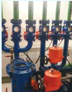
Automatic Tube Cleaning
