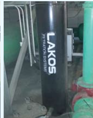
Condenser Water Filtration System
